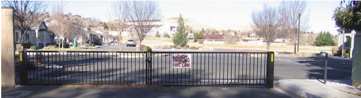
Existing Fence/Emergency Access/Pedestrian Access at Holman Way
